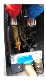
Turn on gas to the water heater, Yellow valve under supply tap cover. The yellow handle aligns with pipe as in photo. Pull grey cover from bottom up.
